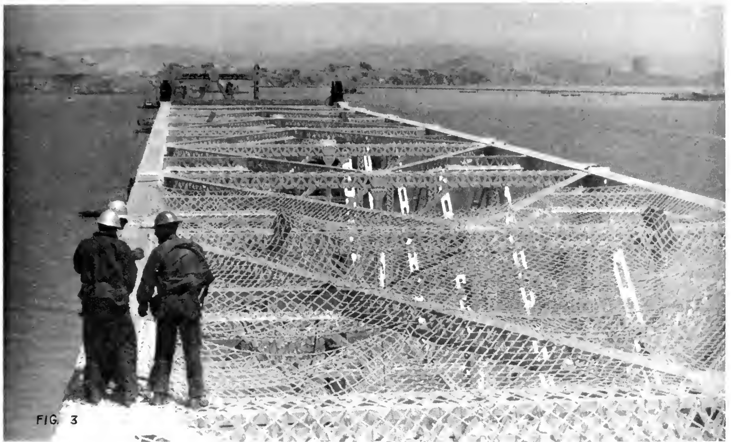
Spreading safety nets on the aluminum span
